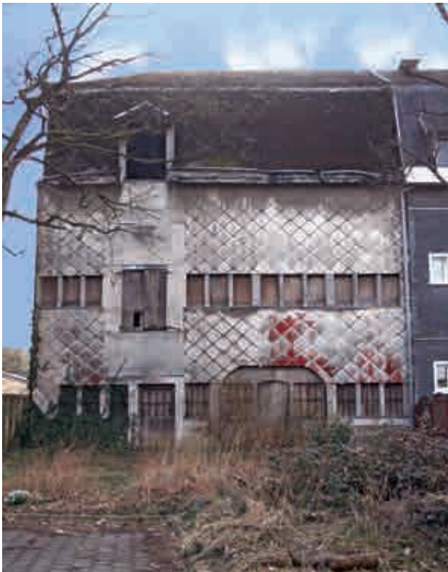
Fig. 21.- Malmedy, la tannerie Kalpers, façade avant. © Alissa Diffels, 2018.
